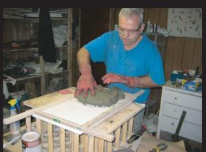
3) Following the prep-work, I create a frame / form to accept the fresh concrete. Armed with previously drawn sketches, I immediately proceed to imbedding the metal pieces into the concrete while at the same time, shaping the metal and the concrete to create the desired shapes. I have a window of opportunity of approximately one hour to complete this step.
